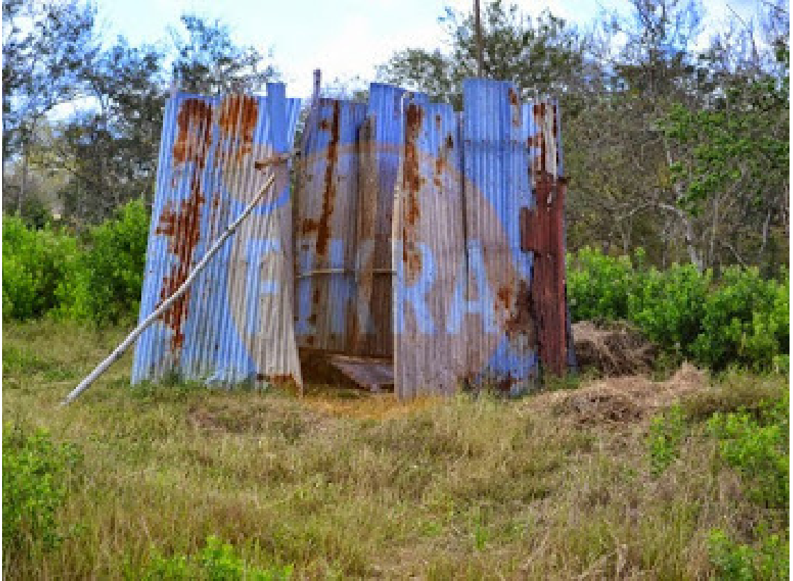
Picture 11: Lavatory at the Kibaha Primary Court
