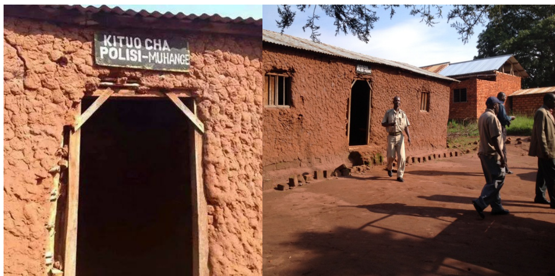
Picture 54: A dilapidated Muhange police post in Kakonko district, Kigoma
