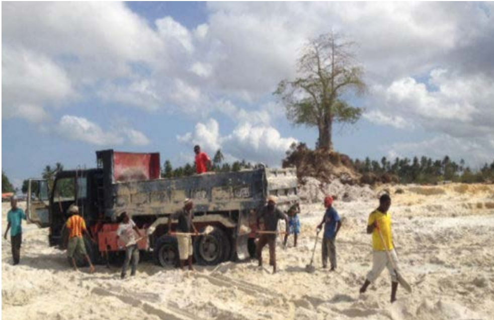
Picture 52: Sand excavation in Zanzibar
