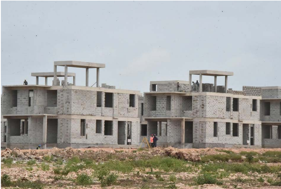
Picture 49: The construction of a new city at Fumba in progress
