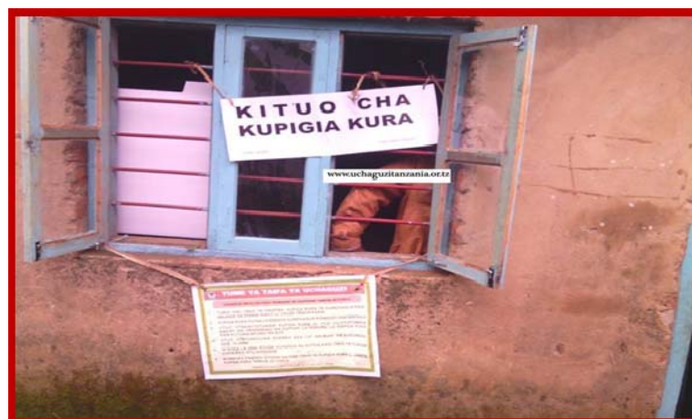
Picture 5.3: A polling station in Bukoba urban hosted in a residential house.
