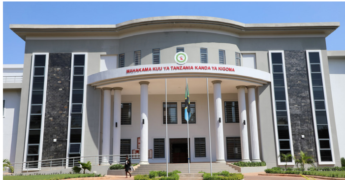
Picture 2: Newly constructed High Court of Tanzania in Kigoma Picture: Judiciary of Tanzania
