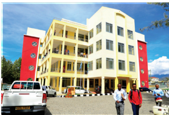
Picture 5: Newly-constructed building at Mzumbe University – Mbeya Campus
