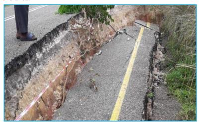
Picture 22: Cracks and potholes due to rainfall damage at Wete Gando Road, Pemba North
