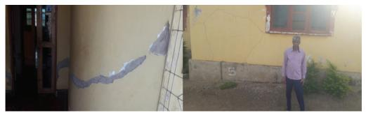
Picture 74: Cracks at the house of one of the villagers of Nyamalambo reportedly caused by GGM mining operations
