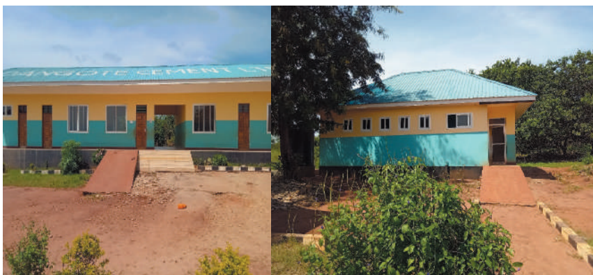
Picture 6.5: Classrooms and toilets constructed by Dangote Cement PLC in Hiari Village
