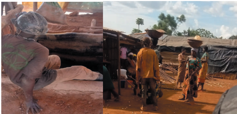
Picture 3.15: Workers (small-scale miners) observed working without PPE at Mwambo wa Luvile Mine in Chato, Gieta
