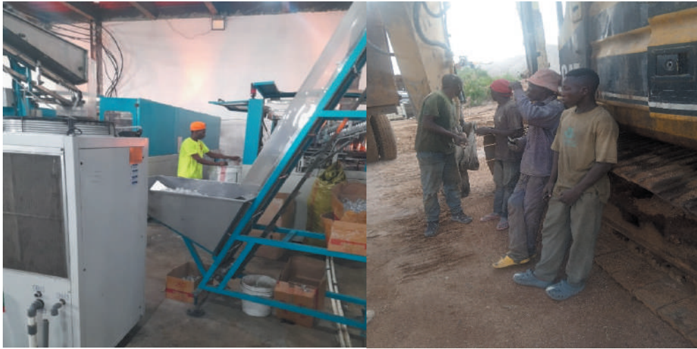
Picture 3.14: Workers observed working without PPE at U-FRESH FOOD Limited in Pwani (left) and Exance Construction Limited in Mara
