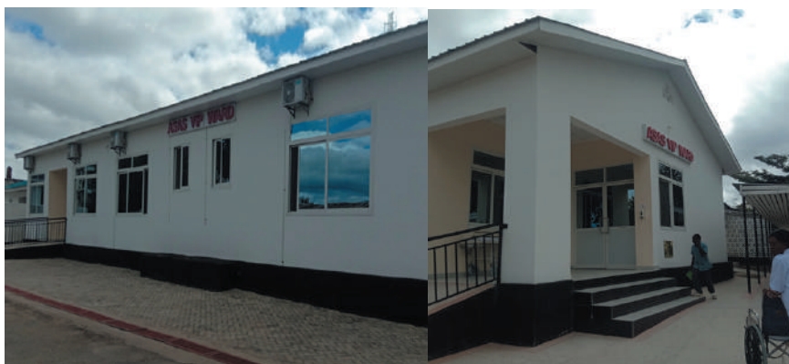
Picture 6.8: A VIP ward constructed by ASAS Company at the Iringa Regional Hospital
