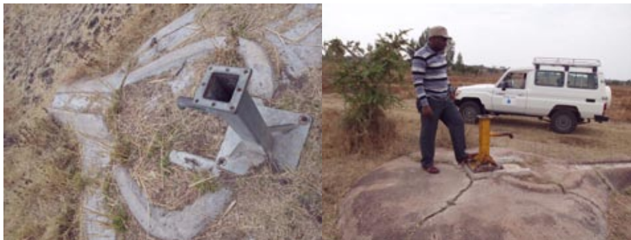
Useless boreholes found in Kwimba District
